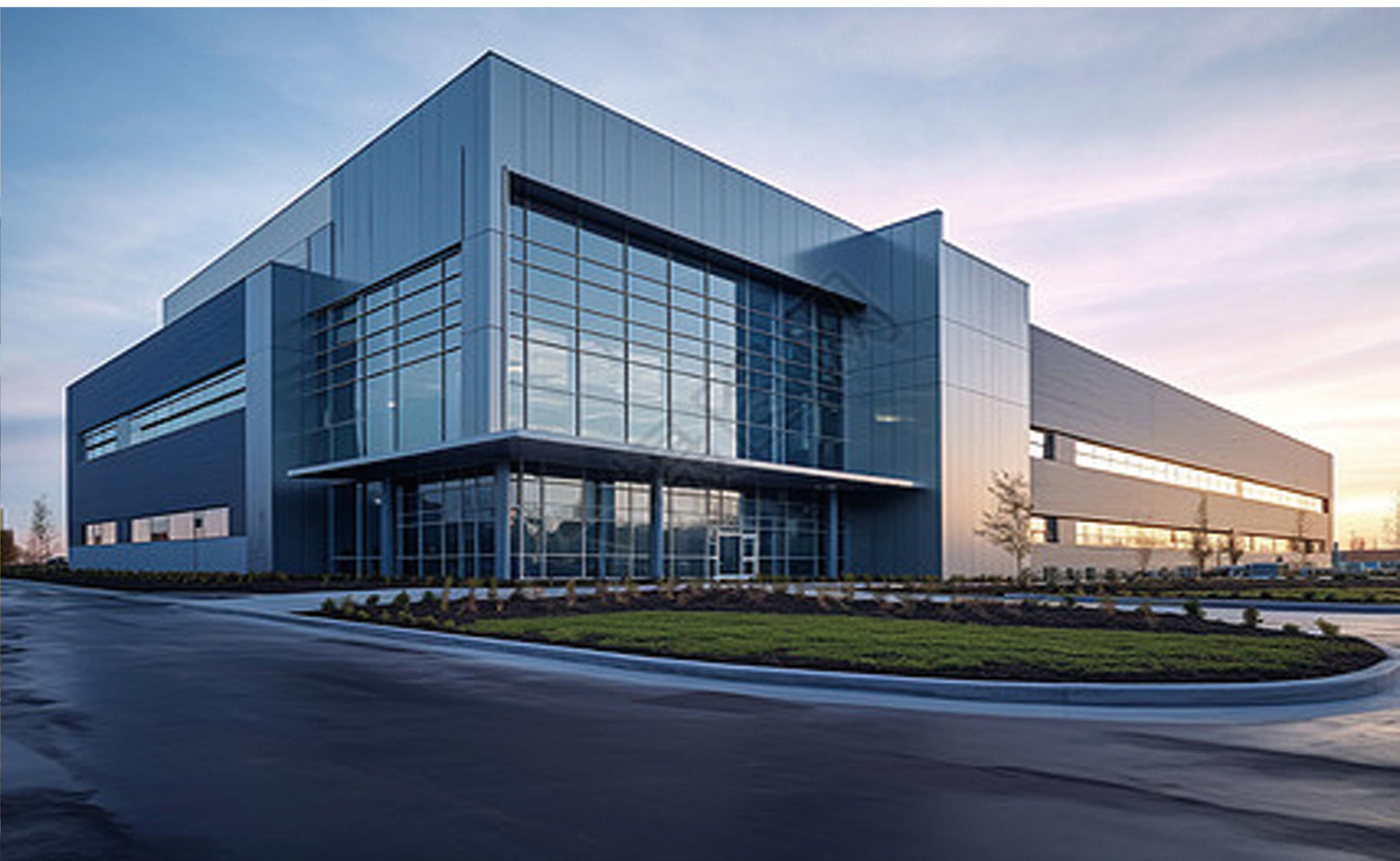
ShanDong plant area (7000m 2 )
